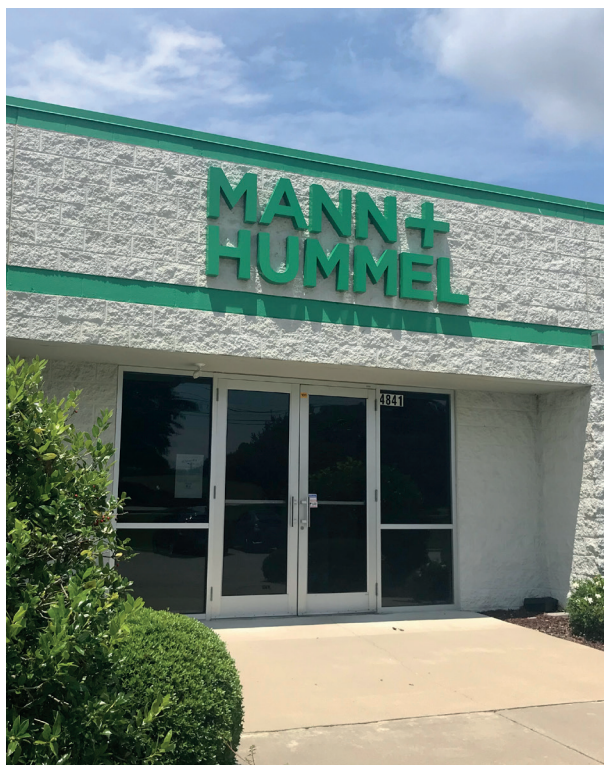
Air Filtration Americas High Purity Manufacturing & Testing Facility Wilson, NC
