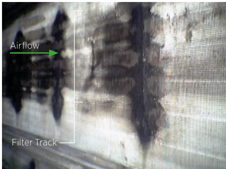
Application photo showing filter track mounted directly in front of the coils.
